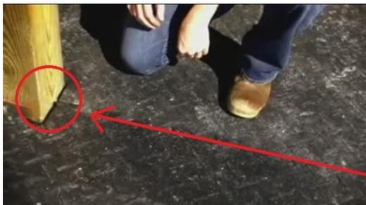
You can place a piece of 2"x4" wood block under the mat (along the place where you need to cut) to help you during cutting
