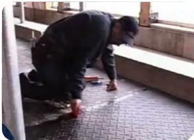
Wipe off any excess sealing material with a scraper or a spatula
