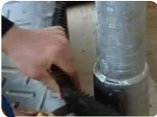
Use a non-retractable knife and cut a notch in the mat in front of the poles
