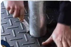
With a hole saw, drill a hole at the end of the cut (where the column will be found).
