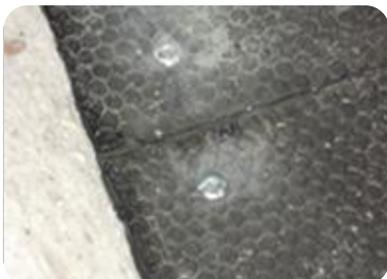
Hammer the anchors in while making sure each one is properly driven into the hole
