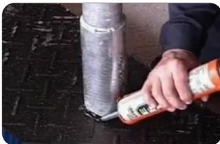
Close the hole and the notch with the sealant
